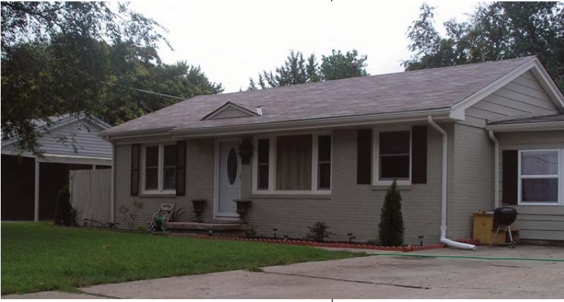
Above, 2008—Eldon & Verda's first purchased home at 201 Alexander Drive in Haysville. The original red brick has since been painted.
